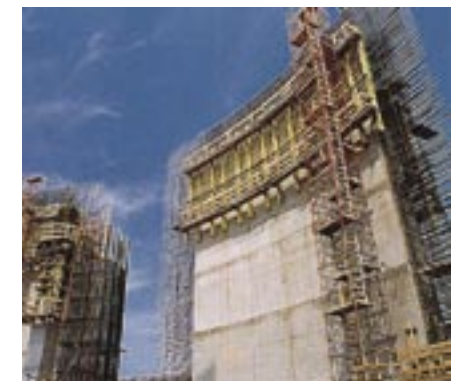
J6 Rocket Test Facility, Nashville
