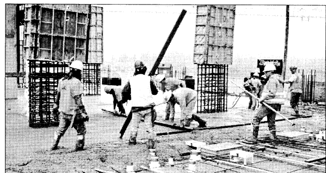
Day 6 – Concrete is poured.
