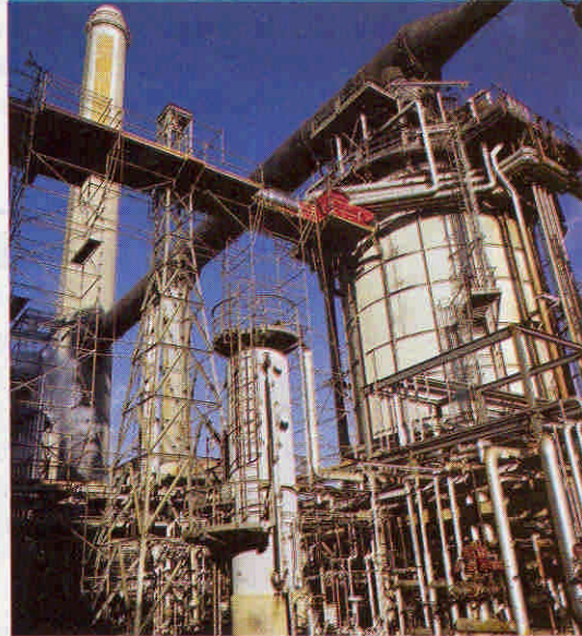
Heavy industrial scaffolding.
