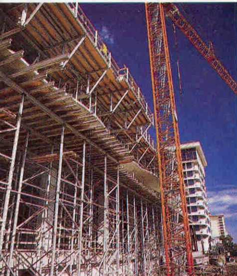
Concrete formwork with Aluma Frames and Aluma Trusses.
