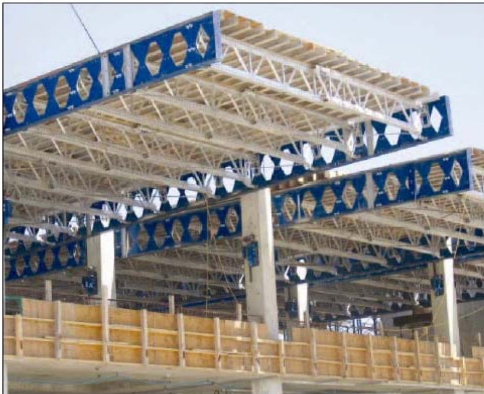
3,000 ft 2 (300 m 2 ) Aluma Hi-Flyer panel put in position.
