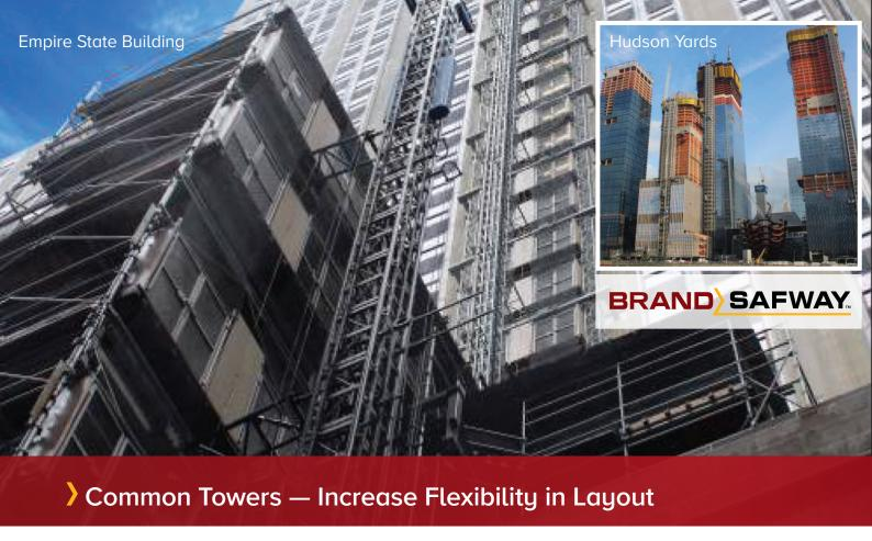
A Common Tower hoist complex uses a temporary "common tower" structure to serve a building with up to 3 dual hoists within a compact and efficient footprint.
