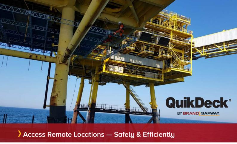
Designed for access challenges in the air, around curves, in tight corners and underneath structures, BrandSafway's proprietary and patented QuikDeck® Suspended Access System improves productivity, reduces costs, saves time and, most importantly, increases safety. A factory floor in the air, QuikDeck allows multiple craftspeople to easily and efficiently
